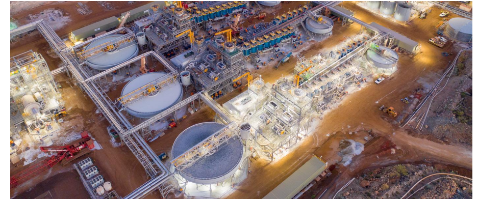
Kemerton Lithium Hydroxide Conversion Plant, WA
