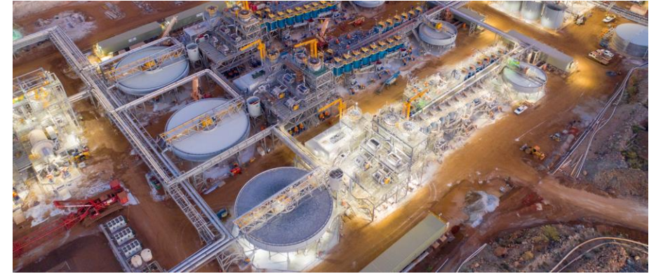
Kemerton Lithium Hydroxide Conversion Plant, WA
